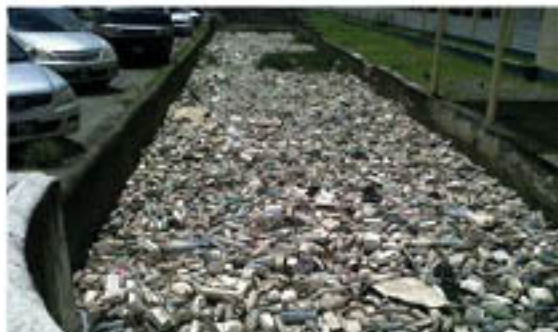
Drain adjacent to a national museum in a CARICOM country on 9/1/14.
